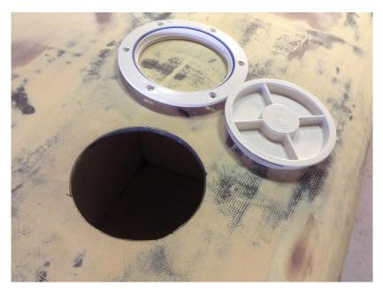
Figure 4.49: Hole for the inspection port.
