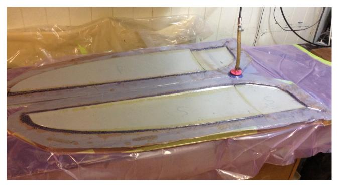
Figure 5.12: Centre-board carbon-HDF sandwich under vacuum.
