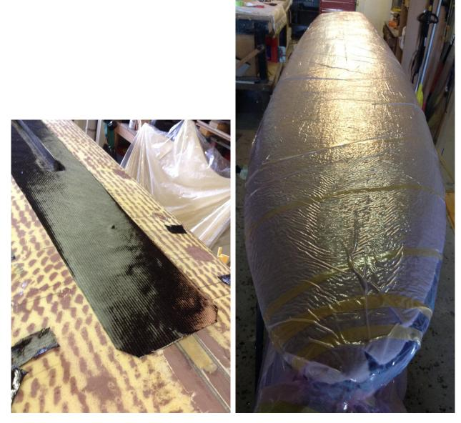
Figure 4.44: Additional patches of  $150 \text{ g/m}^2$  biaxial weave carbon were used on the deck and vacuum bagging  $200 \text{ g/m}^2$  plain weave carbon onto the deck.
