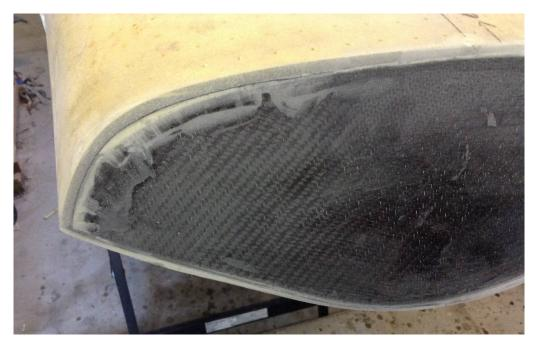
Figure 4.40: Thickened epoxy filler applied into gaps on the stern.
